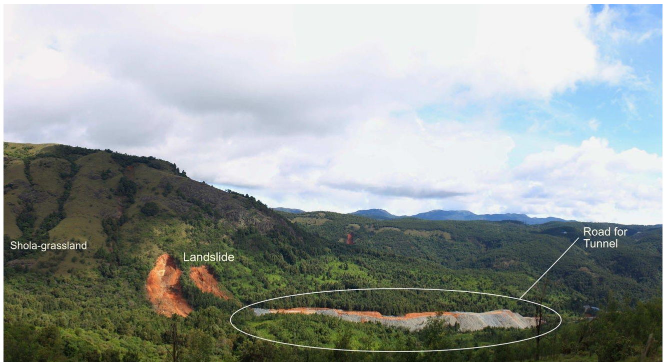
Image 4: Showing a large landslide in a mountain containing shola-grassland vegetation. The landslide abuts a new road construction that services the Kundah PHSEP. Hundreds of these landslides occurred in the monsoon of 2019, in this region.
